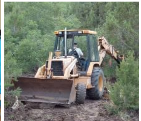
Dale breaking ground on puppy enclosure
