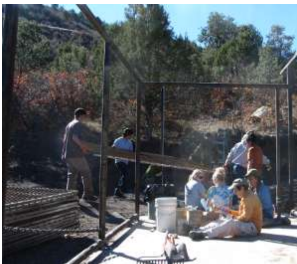
Moving the panels and getting the clamps ready
