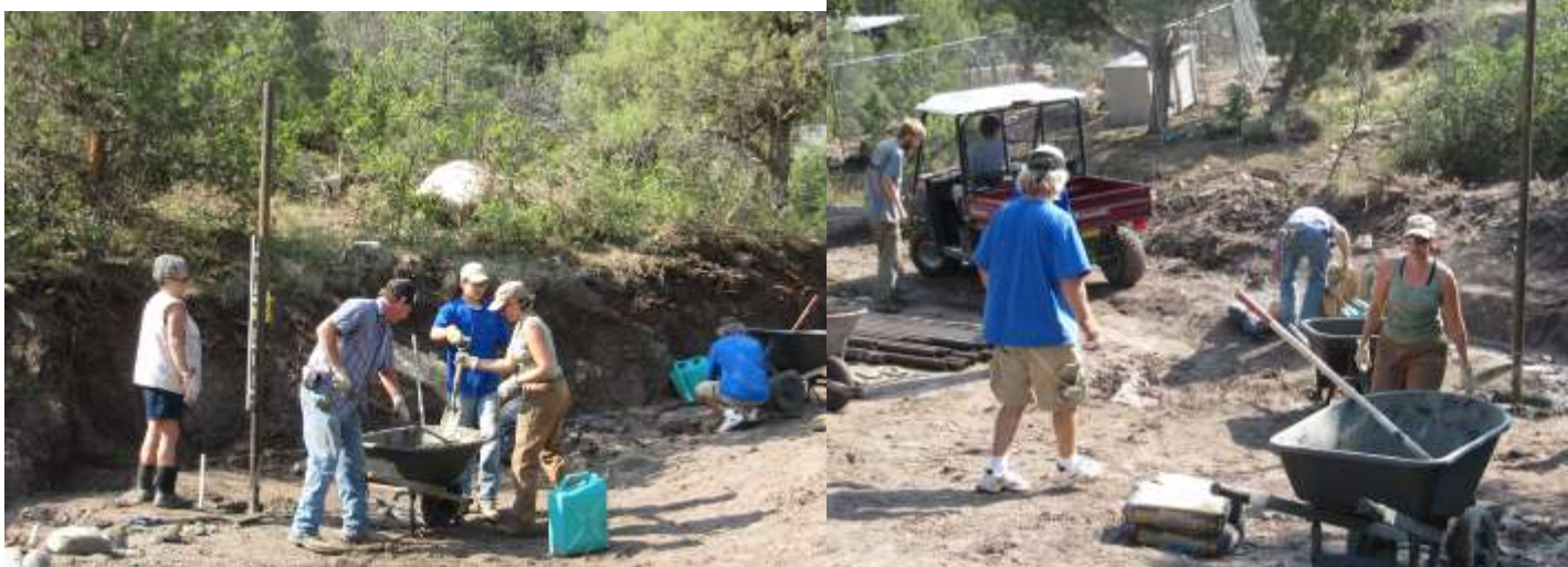
Work crew hauling concrete and setting the poles
