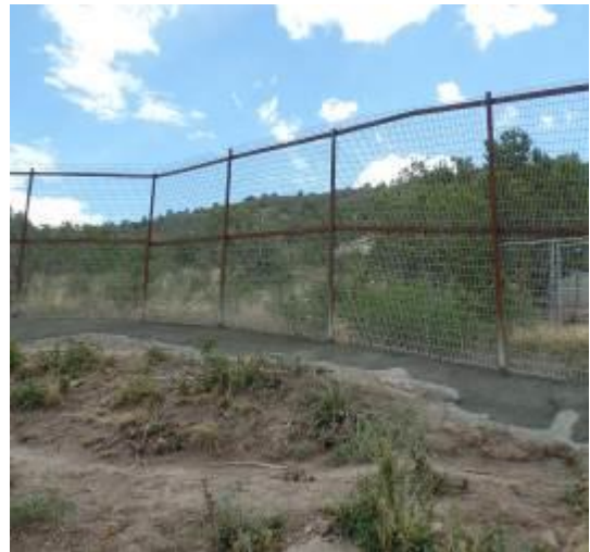
Spraying concrete around Ra and Tala's pen to prevent erosion under the fence line
