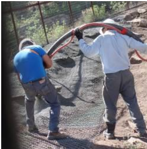
Spraying concrete around Ra and Tala's pen to prevent erosion under the fence line
